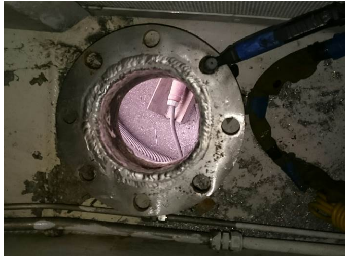
# 3 Before / After but Before Welds Have Been Ground Back
