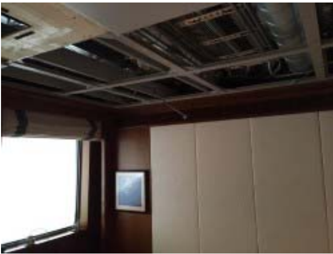
New Cable Runs
