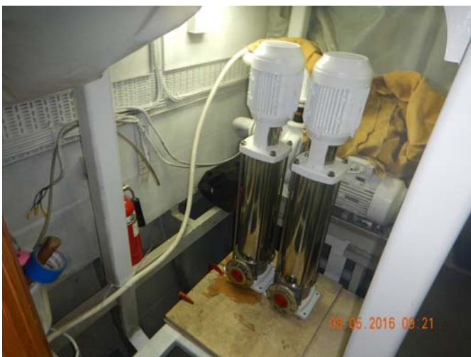
FW Pump Layout for New Piping
