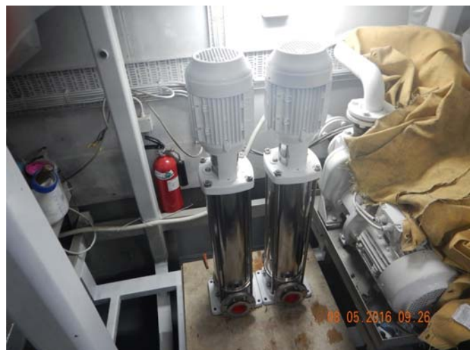
FW Pump Layout for New Piping
