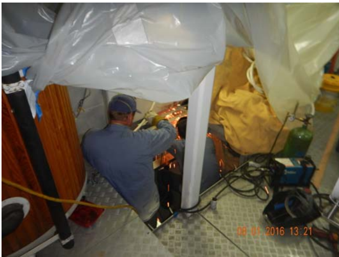
Welding New FW Pump Foundations
