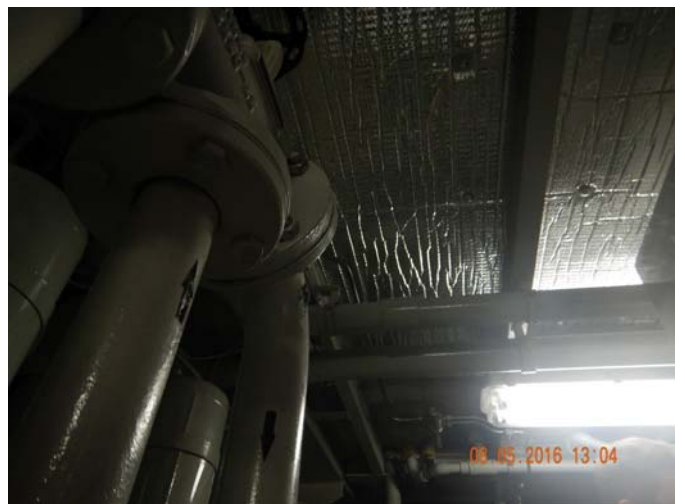
Insulation Install Below Elevator Space
