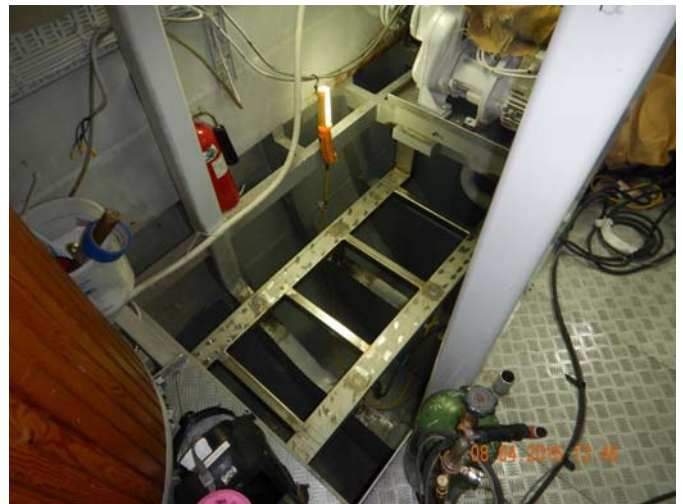
Welding New FW Pump Foundations
