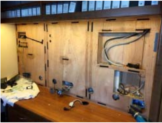
Cutting for New Electronic Install
