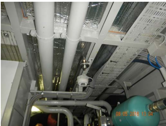
Insulation Install Below Elevator Space
